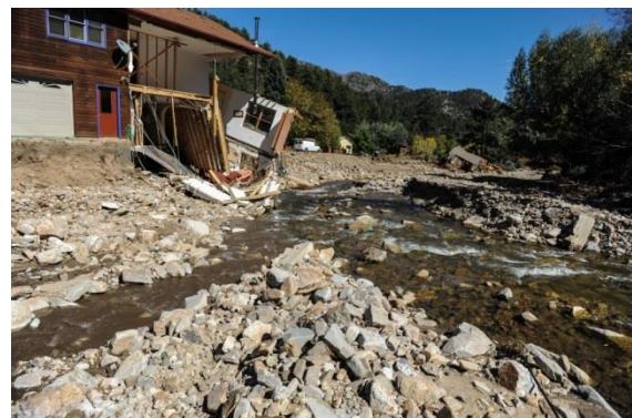
Aftermath of 2013 flood in Jamestown, CO.
