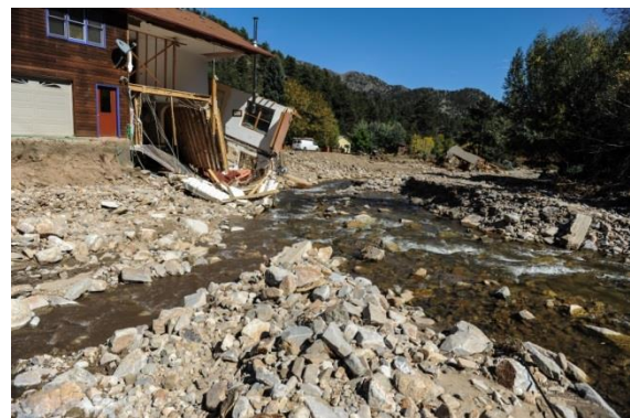
Aftermath of 2013 flood in Jamestown, CO.
