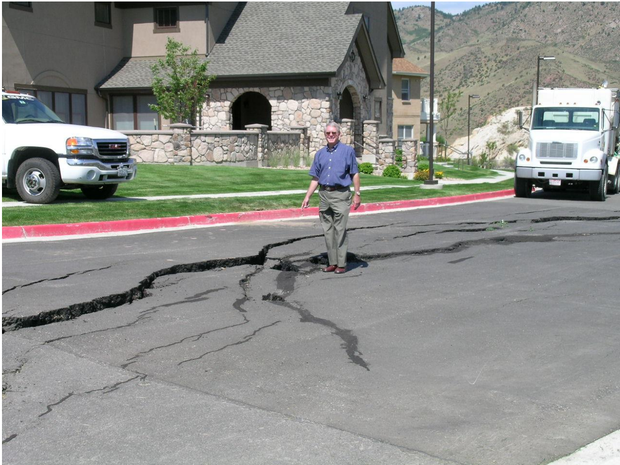
Subsidence is a particular concern for many communities across Colorado. This image from 2005 shows road damage likely initiated by subsidence in Golden near the Colorado School of Mines.
