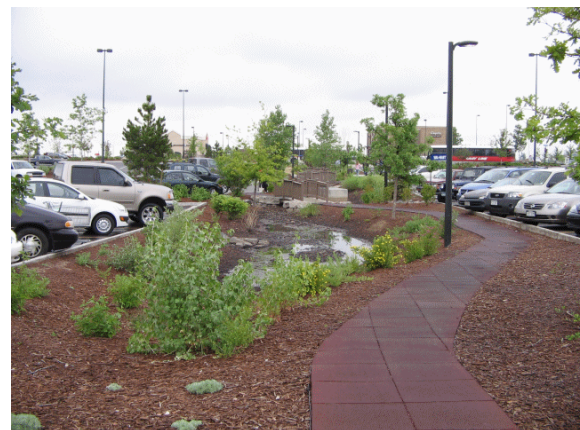
Example of LID (bioswale) in large commercial parking area in Aurora, CO.
